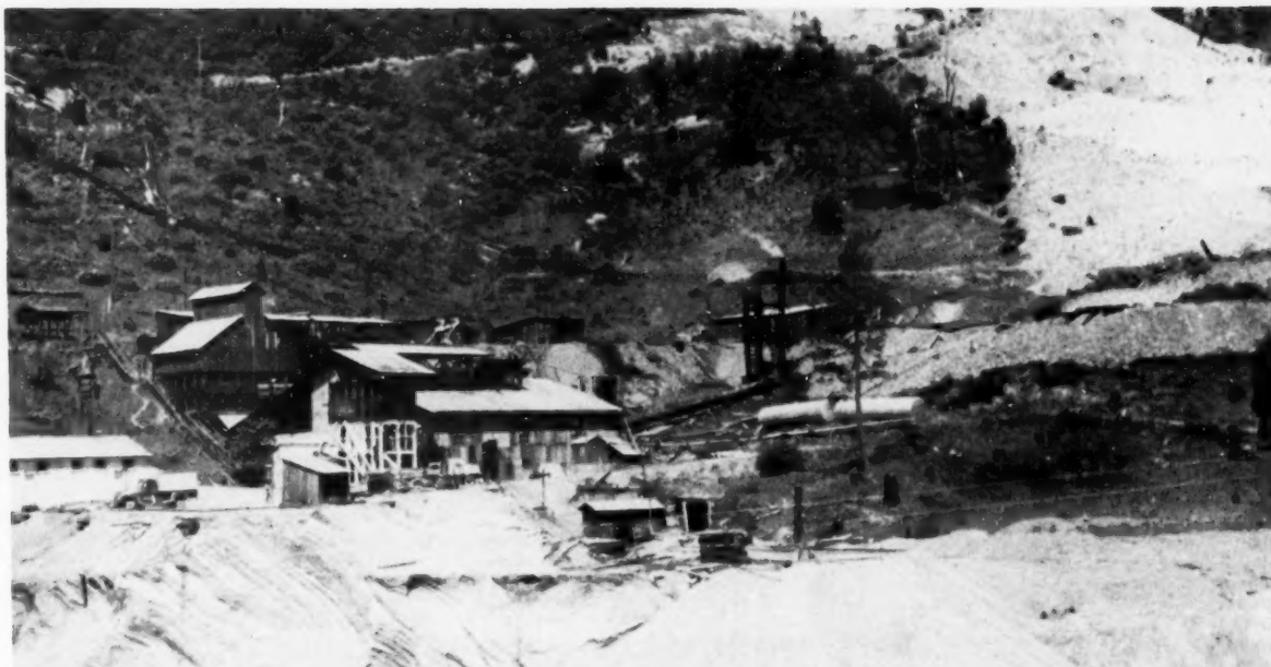
The Bonanza quicksilver mine resumed operations during 1951. Shown here is the mine surface plant near Sutherlin, Douglas County, Oregon. Part of the large calcines dump in foreground.
